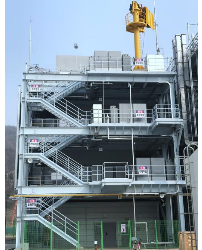
Constrained Space Power Tower 8.35 MW Installation
